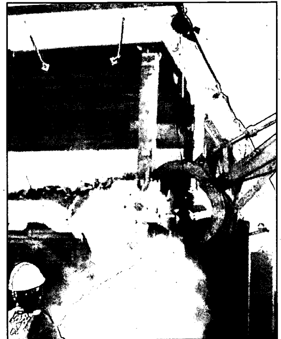
Building 779 demolition work begins in October 1999
