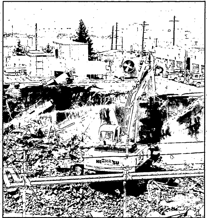
The demolition of buildings at Rocky Flats, such as this one in 1998, will create large volumes of concrete rubble.
