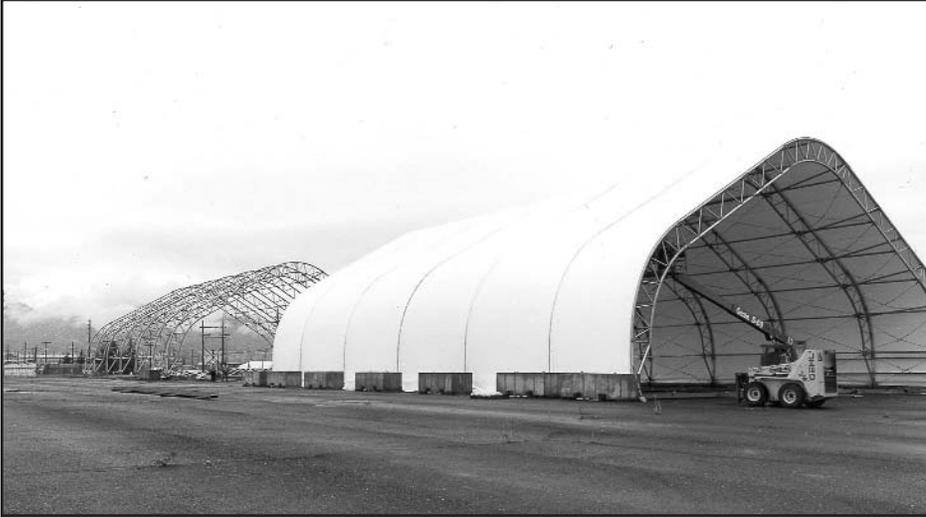
Construction of the protective tent over the 903 Pad is shown above. Work on removal of the asphalt pad began in mid-November.
